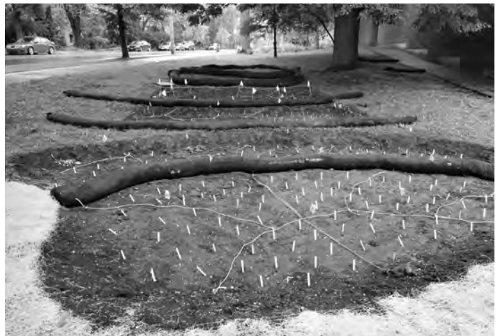
Plant markers and silt socks are installed after the basins are excavated.
