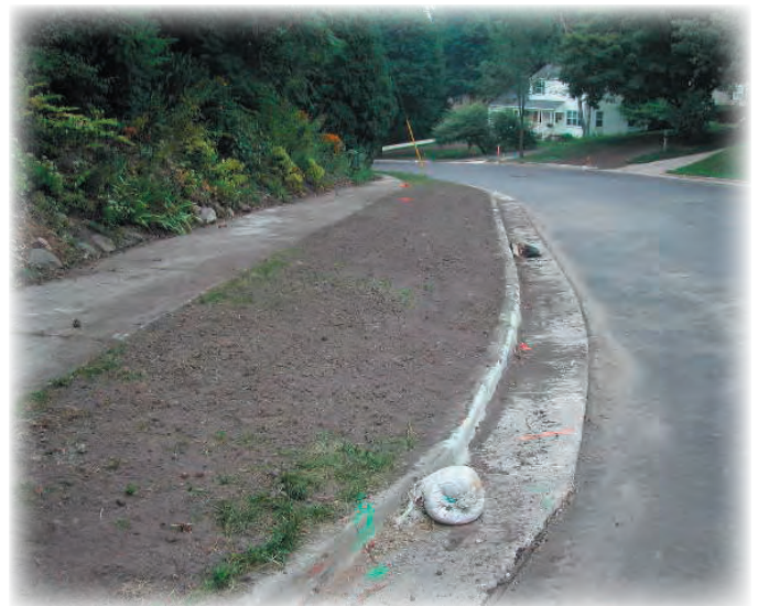
Soil and debris litter this street after construction. If not swept up, all this will go straight into Lake Wingra via the closest storm drain.
