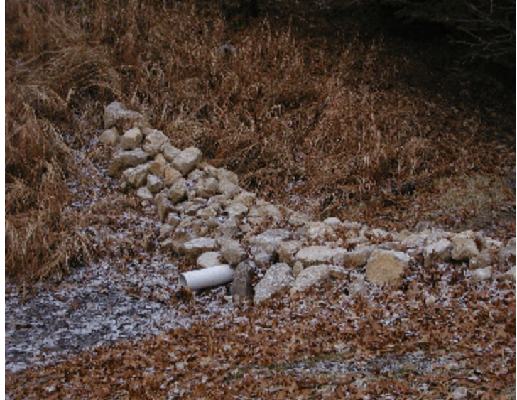
Leyton Lane Check Dam
