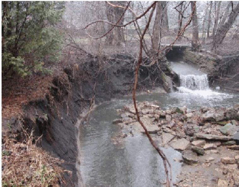
Manitou Way Storm Sewer Outfall
